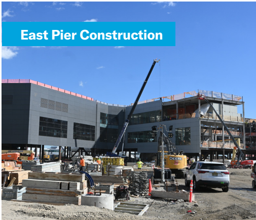
New Terminal One Overview
