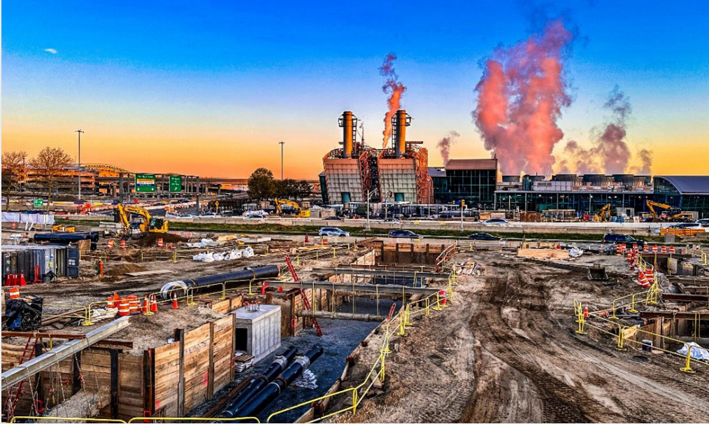
27kV feeders for New CS2 Substation
