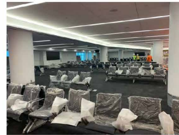
Installing Finishes and Seating
